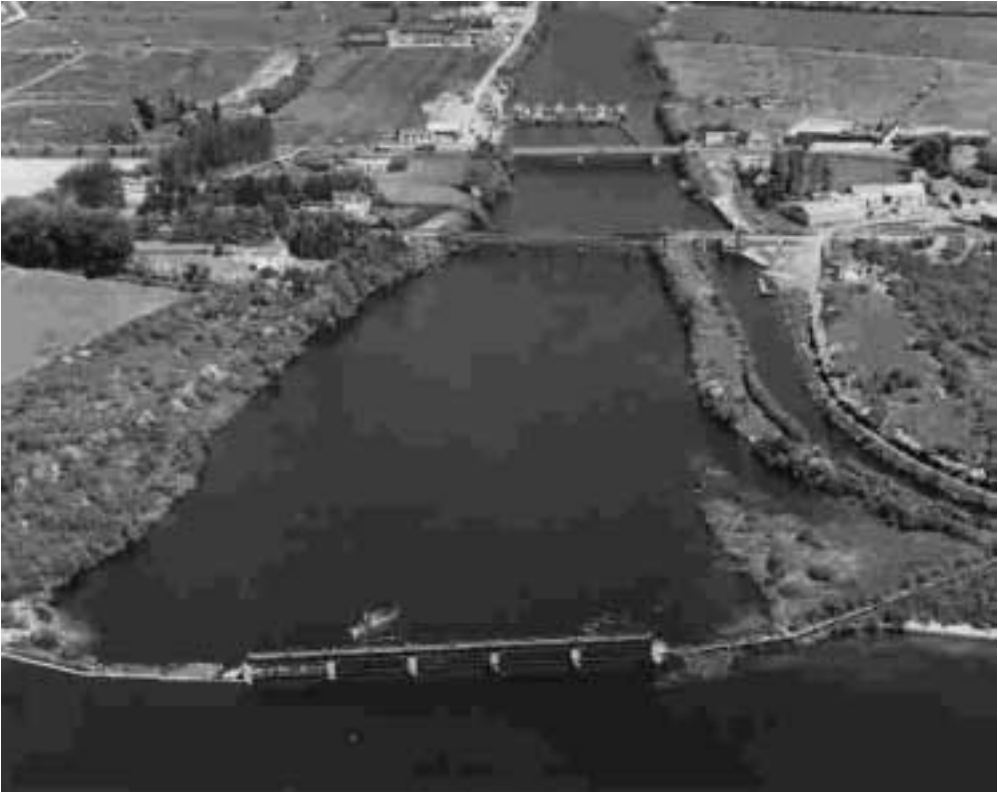
Sluice Gates at Toome.
